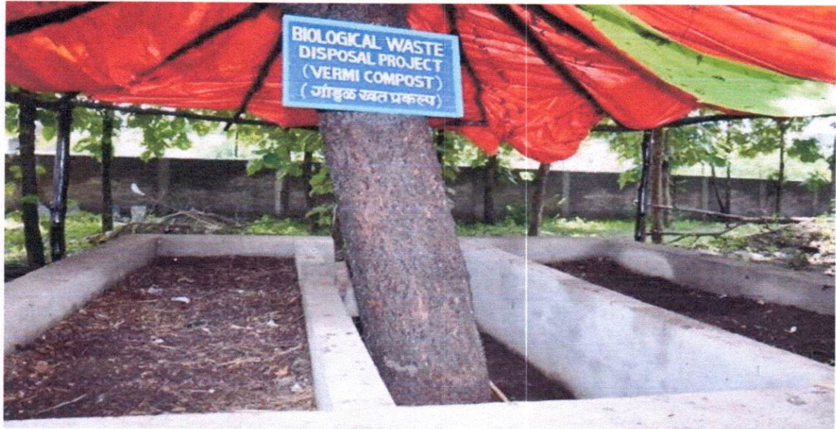
Vermi composting Unit
