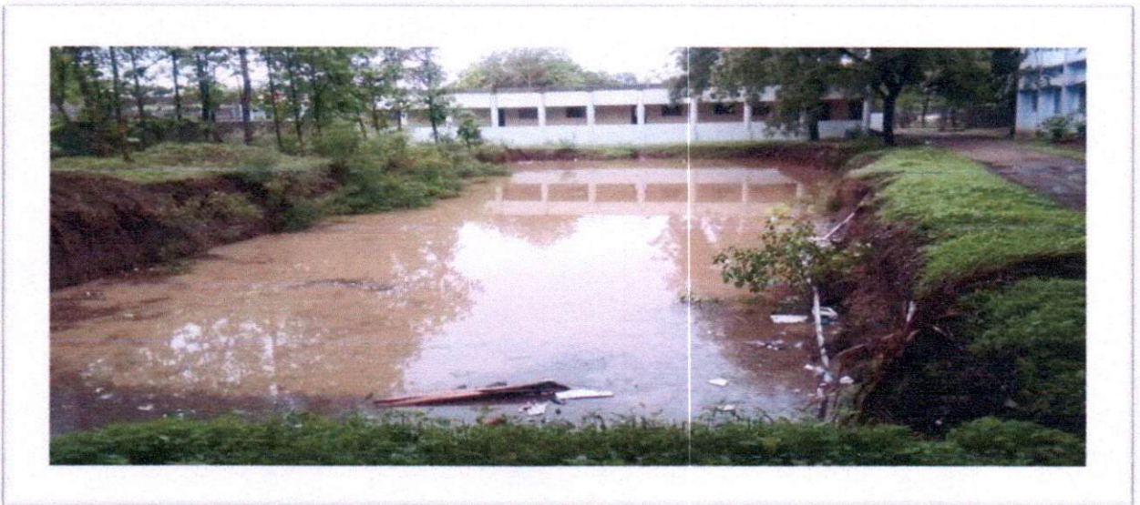
Check Dam Constructed in the campus
